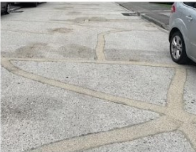
Finished road example
